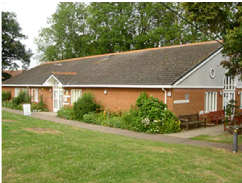
Brambles Surgery — look for this single-storey brick building.
